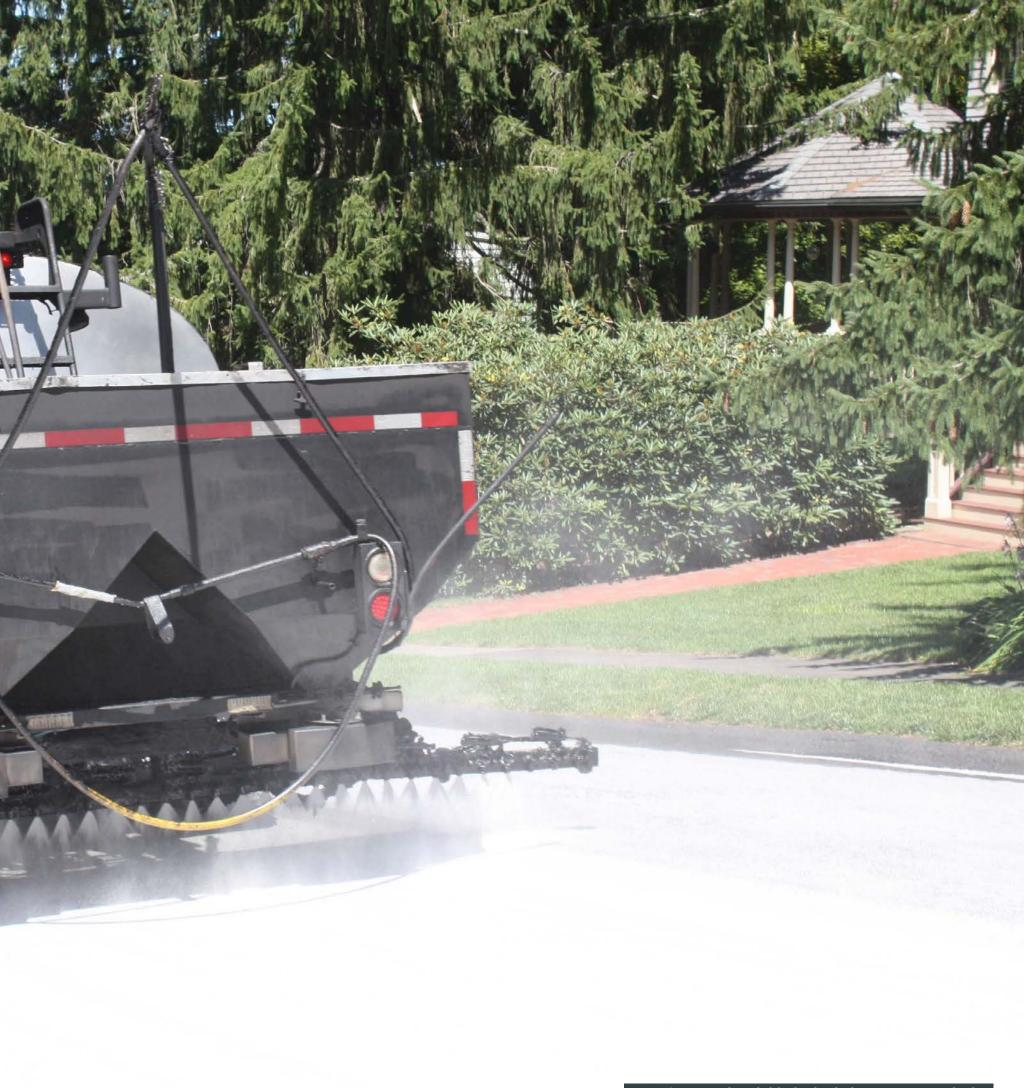
Crews of contractor indus applied the plant-based Delta Mist rejuvenating seal at the rate of 0.08 gallons per square yard at approximately ambient temperature.
